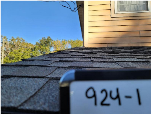
924-1 Asphalt Shingle Typical Exterior Roof
