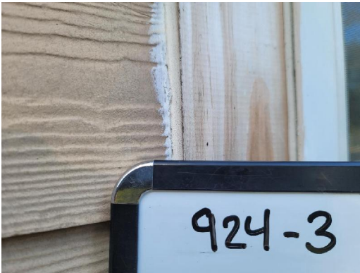
924-3 Caulk Typical Exterior Siding
