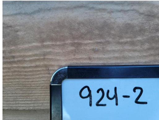
924-2 Cement Board Typical Exterior Siding
